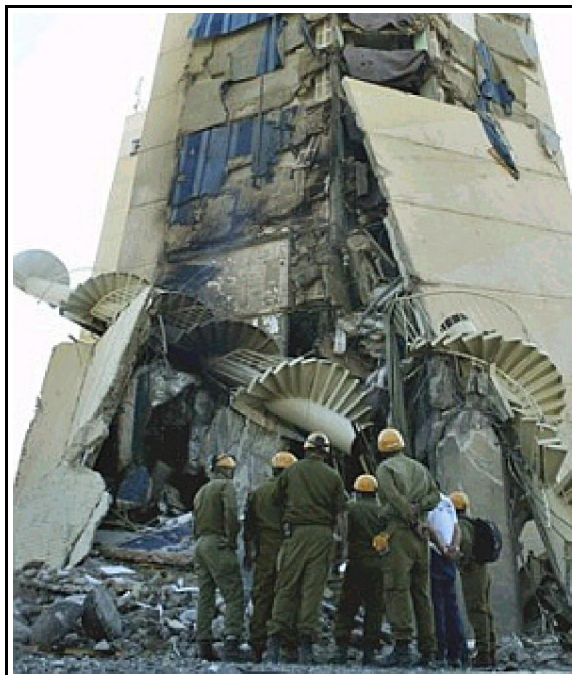
Figure 5 shows the collapsed western wing of the Taba Hilton
